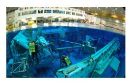
The Neutral Buoyancy Laboratory (NBL) is NASA's astronaut training facility located at the Johnson Space Center in Houston, Texas. The NBL is an engineering marvel. It consists of an indoor pool 202 feet in length, 102 feet wide, 40 feet deep, and contains 6.2 million gallons of water. That's 23.5 million liters for you scientists and Europeans! The pool is used to train astronauts for spacewalks in upcoming missions. The NBL contains full-sized mock-ups of the International
